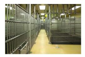
Full-size mockups of pens and gates were built and tested to ensure maximum safety, with quick escape routes for handlers, latches that animals could not learn to operate, and strong, flexible materials with no protruding sharp surfaces or pinch points. (*Photo courtesy of Merrick & Company.*)
