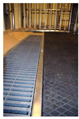
The channel-cut, grooved, rubberized flooring system in use at the Ames facility directs water toward drains, eliminates the need for animal bedding, and absorbs noise. (*Photo courtesy of Merrick & Company.*)
