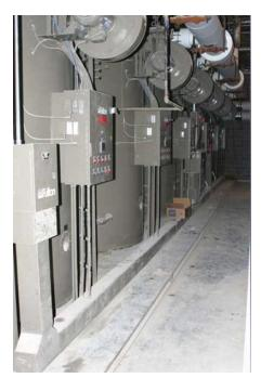
The BRI features dual electrical feeds, three chillers, a 2000-kw backup generator, and a 10,000-gallon fuel tank with a 14-day reserve to support biocontainment operation of the building. (*Photo courtesy of Scott Rusk,* Kansas State University.)
