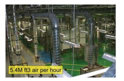
Six independent air handling systems supply various parts of the BRI at Kansas State University. There are 131 HEPA filter housings and the air systems circulate about 5.4 million cubic feet of air per hour. (*Photo courtesy of Scott Rusk, Kansas State University.*)
