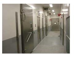
K-State's Biosecurity Research Institute has 21 compression seal gastight doors and nine air gasket sealed doors. (*Photo courtesy of Scott Rusk, Kansas State University*.)
